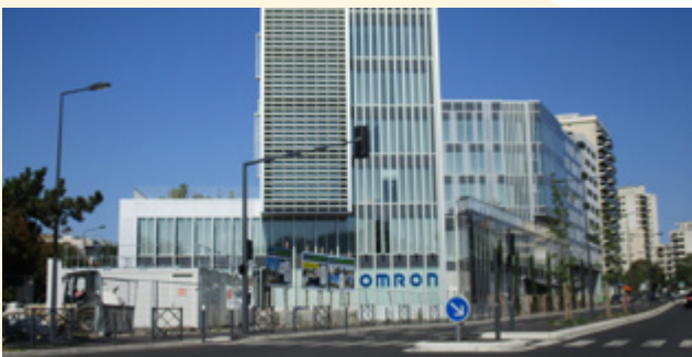
Immeuble Be Office SCPI Carac Perspectives Immo
