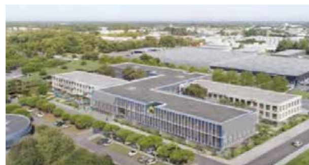
Immeuble Mérignac SCI Community Invest
