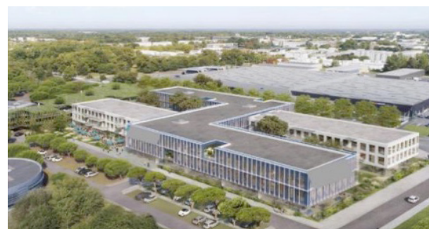
Immeuble Mérignac SCI Community Invest
